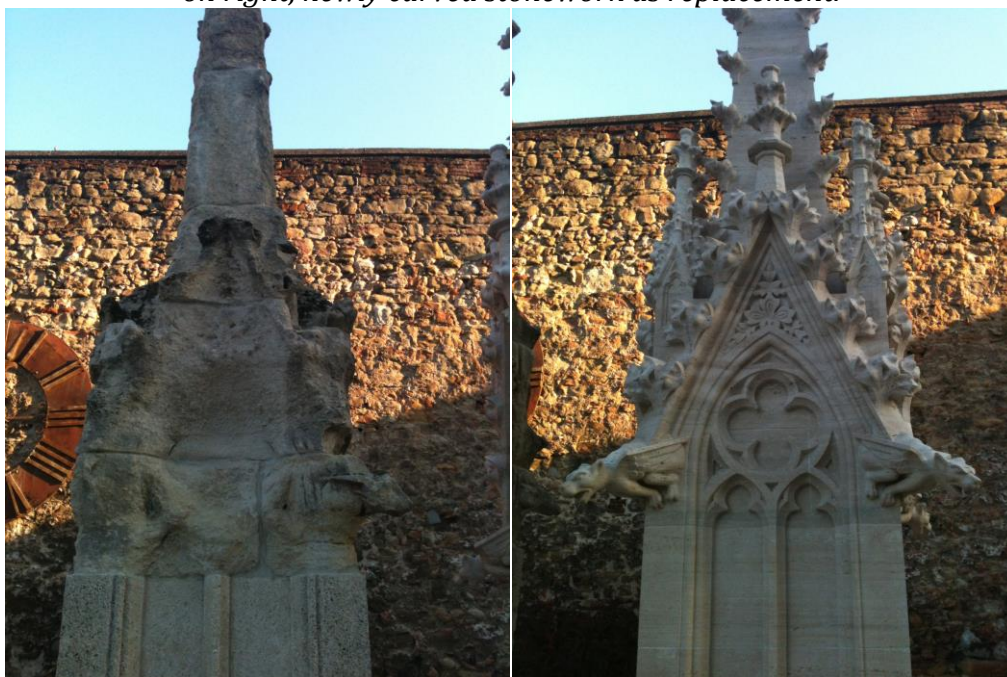
Figure 2. Damage to stonework at Zagreb Cathedral, Croatia, from acidic deposition. On left, the original stonework showing the decay after reconstruction at the end of the 19 th century, on right, newly carved stonework as replacement.
